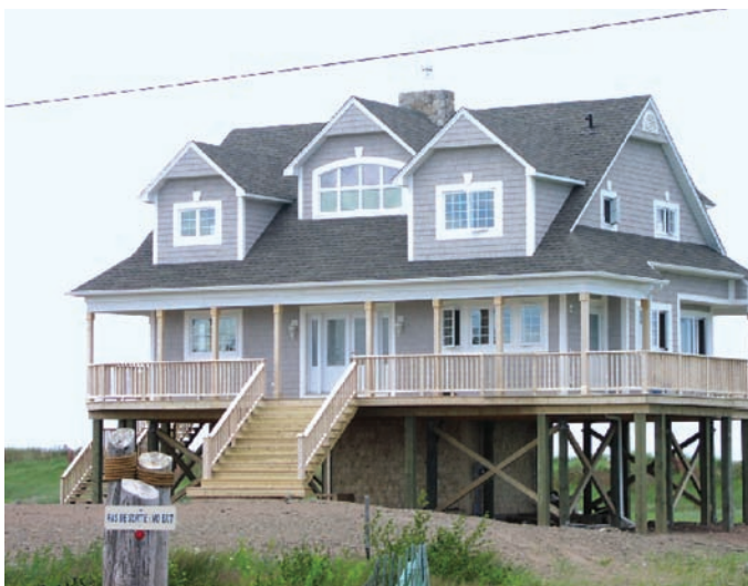
FIGURE 18: Construction of buildings on pylons as an example of adaptation that reduces vulnerability to storm surges, Grand-Barachois (near Shediac), Northumberland Strait, southeastern New Brunswick. Photo courtesy of Armand Robichaud.
